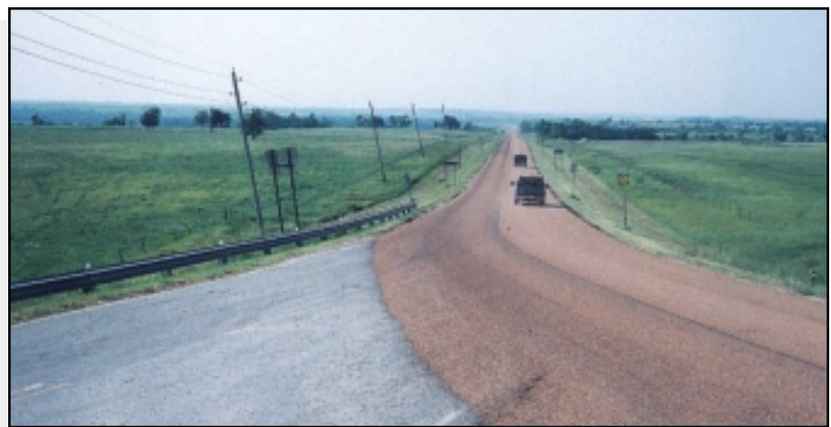
Kansas Hwy.15. Left side is 4 days old. Right side is 2 hours old.
