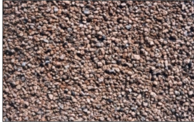
Close-up view of LITE-WATE. 1-hour-old placement. CRS-1 HP @ 0.38 gal/sy. LITE-WATE @ 120 sy/cy
