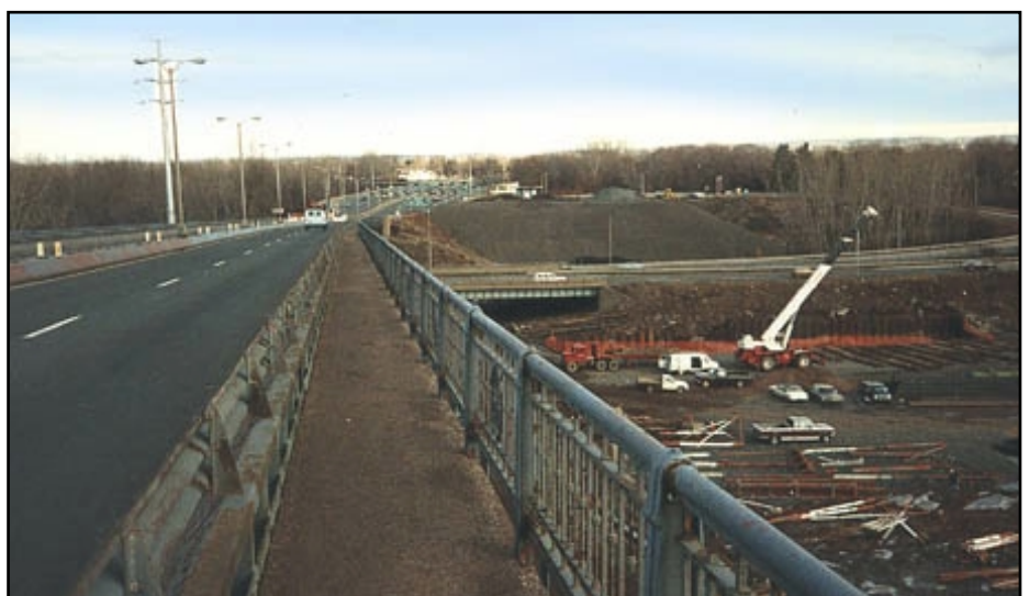
Lightweight fills at east side of river
