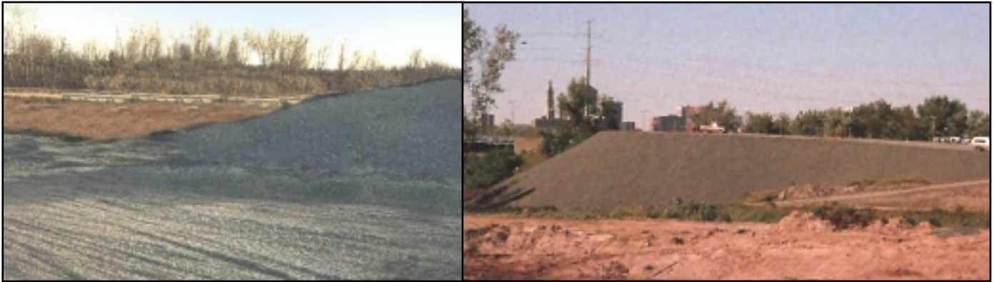
Progress of lightweight fill
