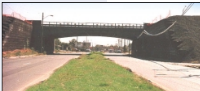
Lightweight fill at approach area
