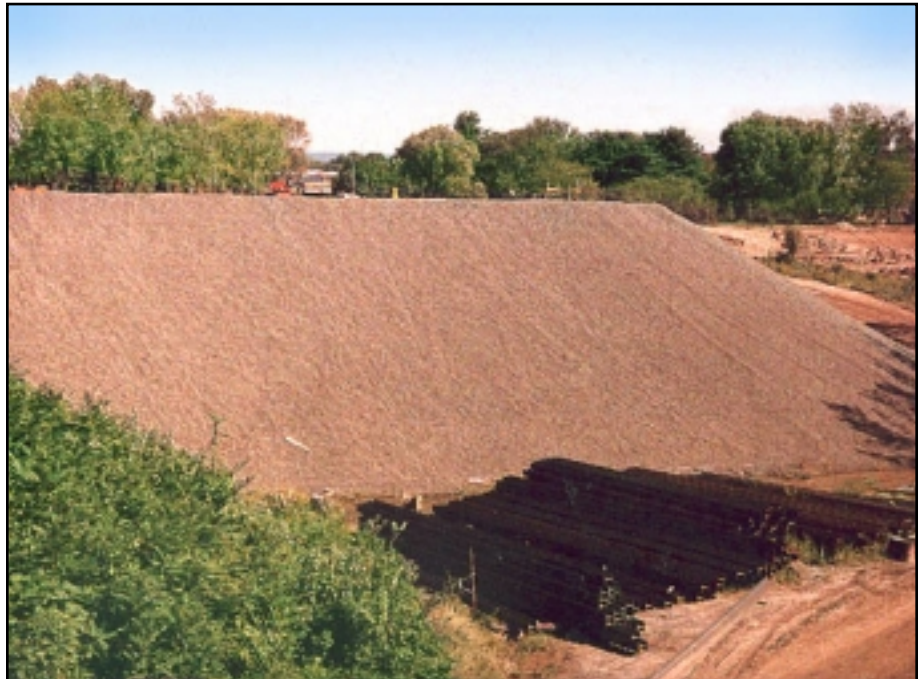
Progress of lightweight fill at east abutment
