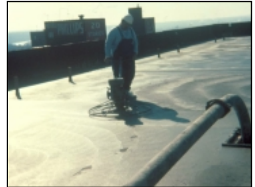
Worker making first pass over lightweight concrete with walk-behind power trowel.
