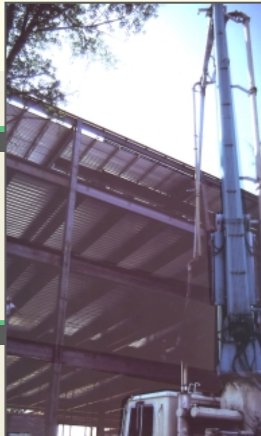
Pumping Structural Lightweight Concrete on Steel-Frame Construction
