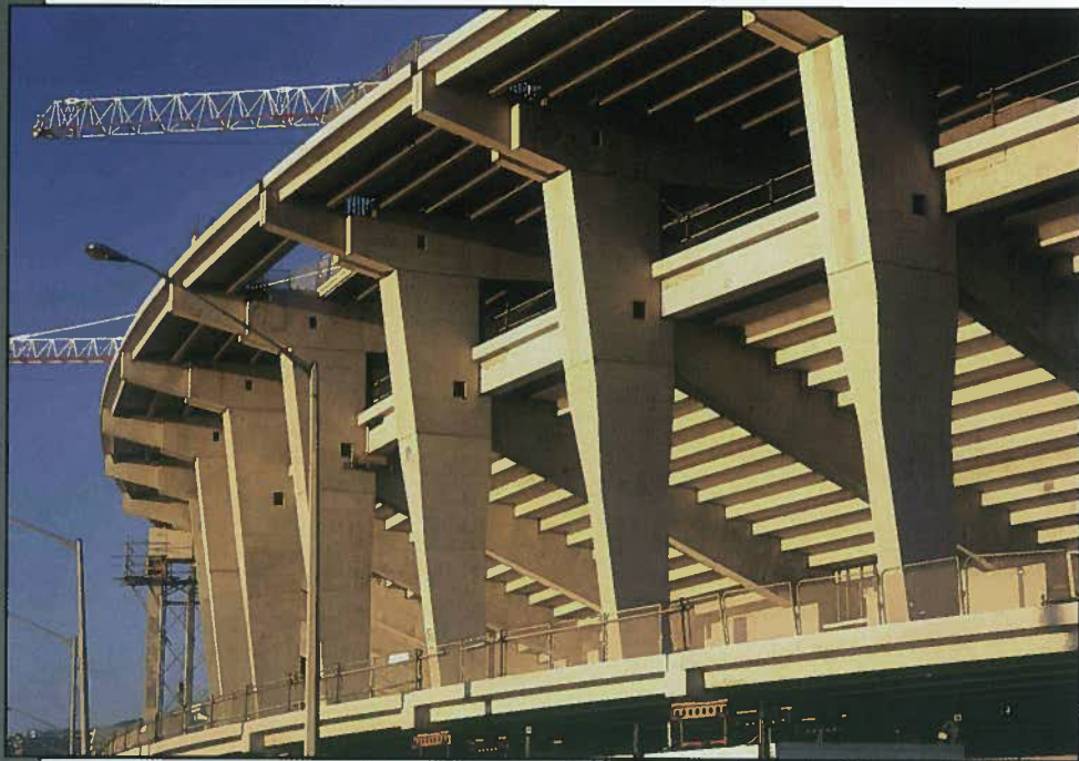
Exterior of 40,000-seat Wellington Stadium nearing completion
