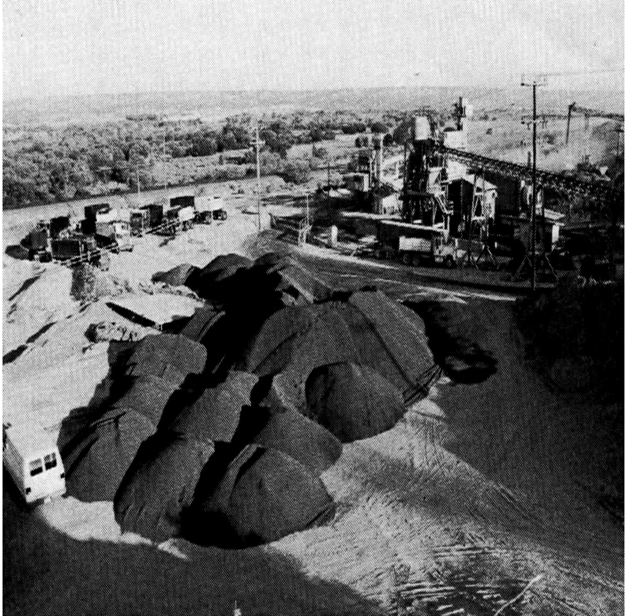
Figure 14.25 Prior to the start of the I-15 job, the ESCS (Baypor) ESCS aggregate was stockpiled at the Industrial Asphalt hot plant in Oro Grande, California. The aggregate was precoated at the rate of 2.5 to 3.0 percent by weight of lightweight aggregate with AR-4000 paving asphalt. It was then loaded into end dump trucks for about a 12 mile (19 km) trip to the jobsite.
