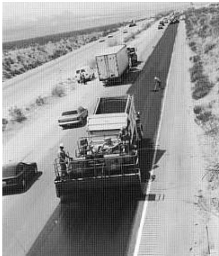
Figure 14.27 I-15 Asphalt-rubber chip seal project showing chip spreader.
