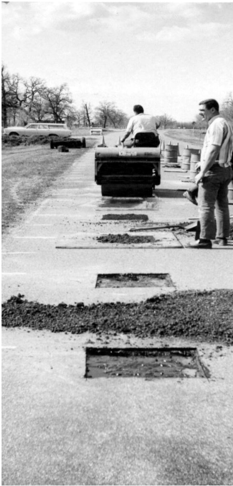
Figure 14.22 Hot-mix cold-lay patching material made with ESCS aggregate
