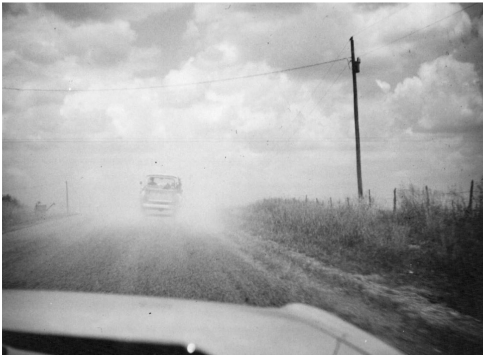
Figure 14.14 Dust caused by steel-wheeled roller use.
