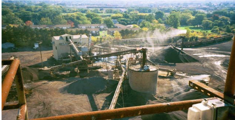
Figure 2.9. Aerial View of Plant
