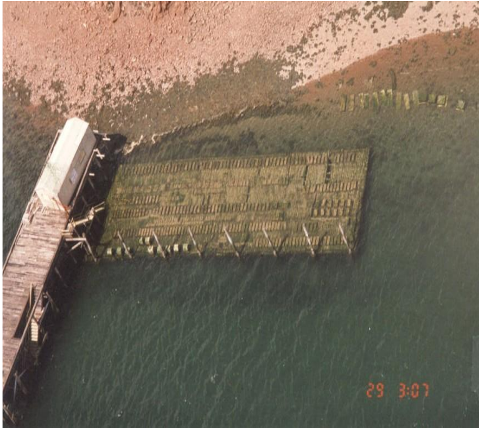
Figure 8.10 Treat Island, Maine research center Lightweight concrete specimens in bottom row. Exposed To two tidal cycles per day (R. Holm, 1998)
