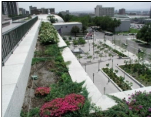
Perimeter planting on roof of LDS Conference Center in Salt Lake City, UT.
