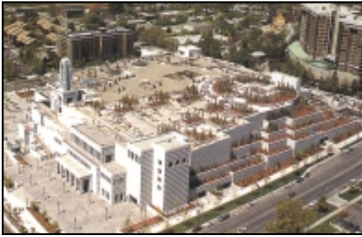
7-acre rooftop garden atop LDS Conference Center in Salt Lake City, UT.
