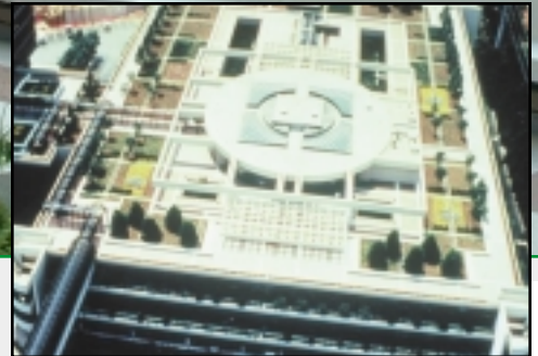
(Inset) Aerial view of North Park roof after installation in 1997
