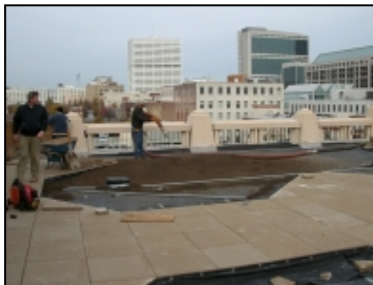
SOILMatrix installed by blowing equipment atop six-story Atlanta City Hall
