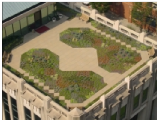
Extensive greenroof garden, City Hall, Atlanta, GA, 2004
