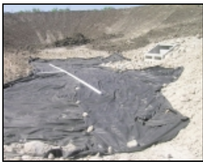
Jordanelle Ridge, Heber City, UT, Storm water rain basin under construction
