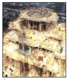
Concrete was pumped more than 750 feet to top the tower.
