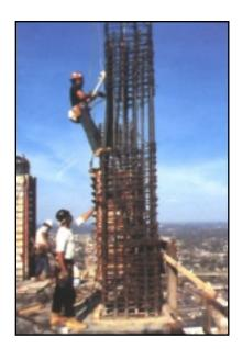
Extra ties were required on column reinforcing to meet seismic requirements. Tower's floor slabs and floor beams were formed of 5,000 psi lightweight concrete.
