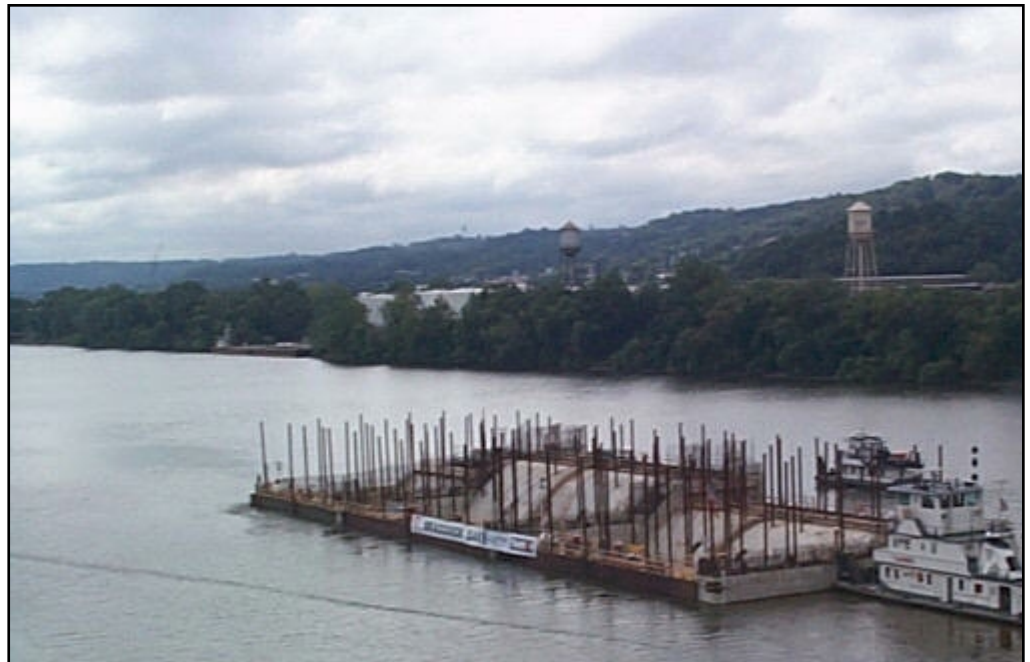
Floating dam Section # 1 being transported up the Ohio river
