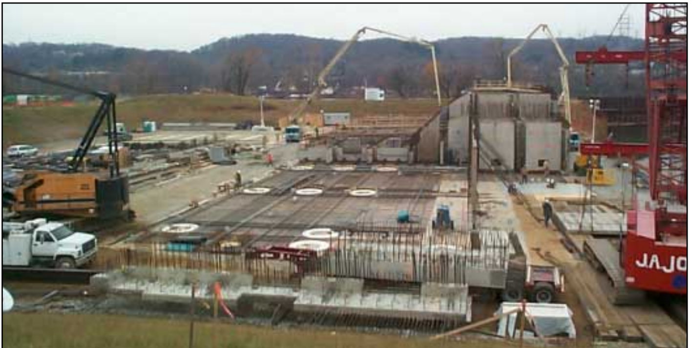
Dry dock construction
