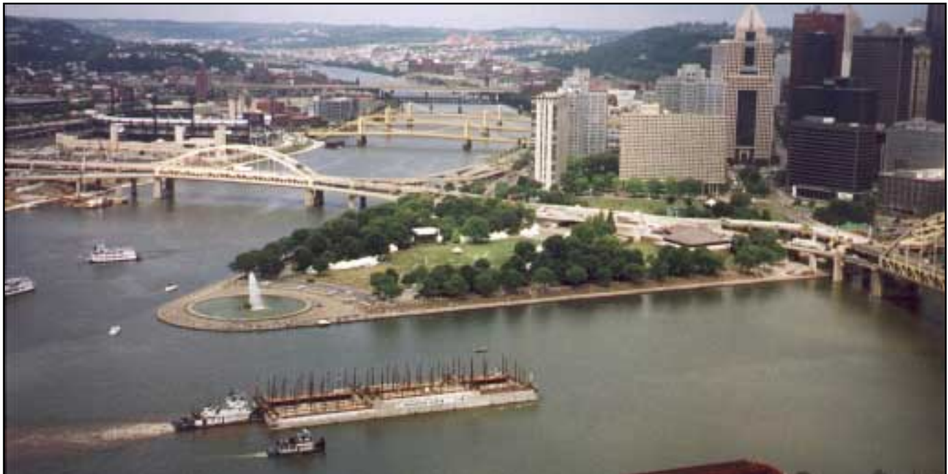
Dam Section # 1 passing downtown Pittsburgh on the Monongahela River
