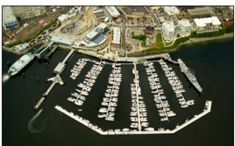
A 1,440 foot-long floating concrete breakwater was constructed in the state of Washington using TXI Expanded Shale & Clay fine graded lightweight aggregate produced at TXI's Boulder, Colorado facility. The \$8 million breakwater project was designed for the Port of Bremerton Marina to attenuate wind driven waves and ferry wakes. Additionally, it was designed to upgrade the marina's boat capacity, and enlarge the waterfront public space extending from an upland public park area.
