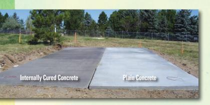
Internal Curing using prewetted expanded shale, clay or slate (ESCS) lightweight aggregate is a simple and practical way of supplying additional curing water throughout the concrete mixture. This is done by replacing some of the conventional sand in the mixture with an equal volume of prewetted ESCS fine aggregate. IC is often referred to as "curing concrete from the inside out."
