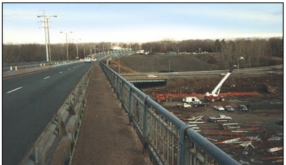
Lightweight fills at east side of river
