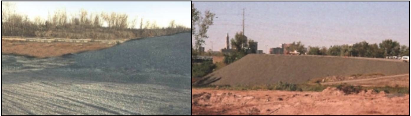
Progress of lightweight fill
