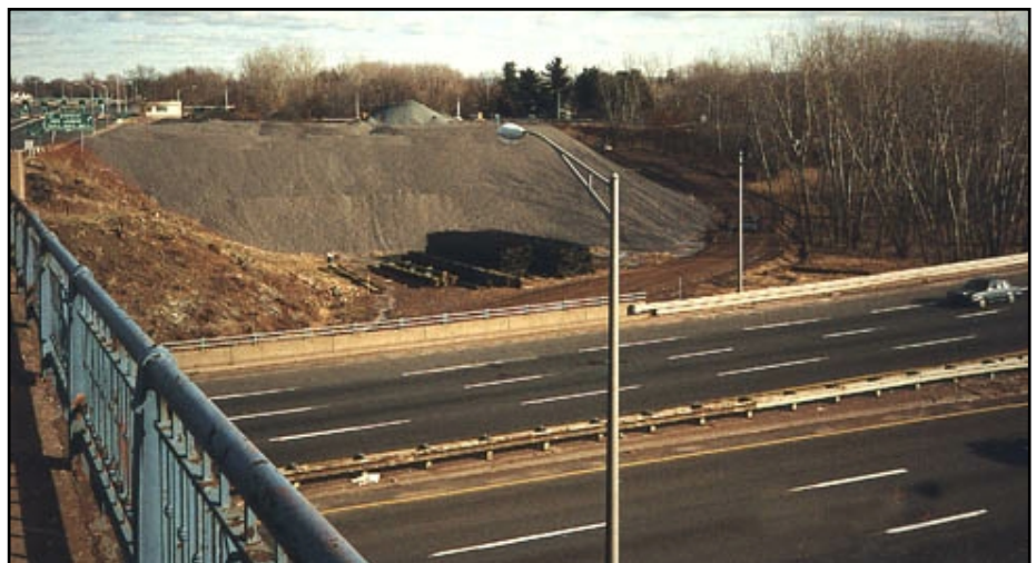
Lightweight fill at east abutment
