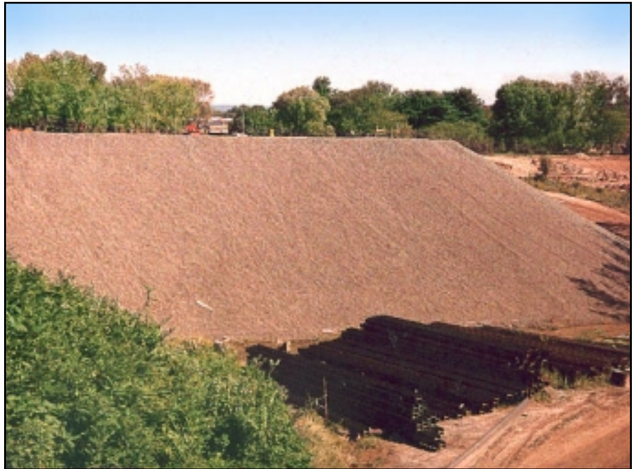
Progress of lightweight fill at east abutment
