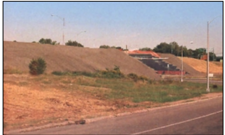
Lightweight fill at approach area
