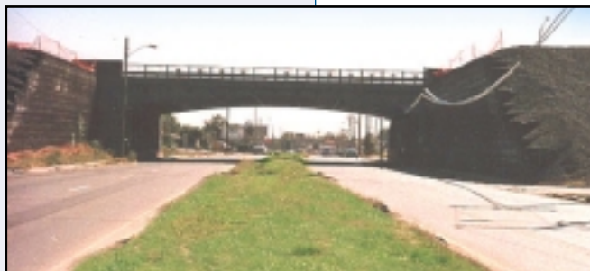
Lightweight fill at approach area
