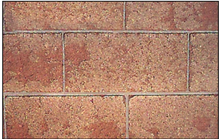
After 4-hour lab fire test at 2,000°F, examination of this walls shows that the CMU's are essentially unchanged except for thin surface damage.
