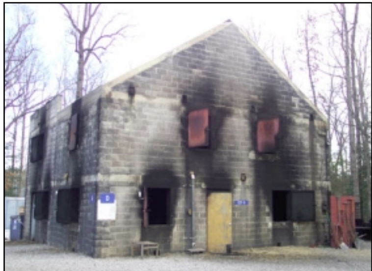
After 25 years and 6,000 fires, the "burn building" looks damaged, but is actually as structurally sound as when it was new.
