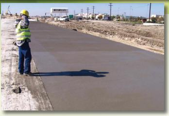
water throughout the concrete, so more of the pores remain water-filled, minimizing stress and strain development. This reduces or eliminates early age cracking of the concrete and promotes
