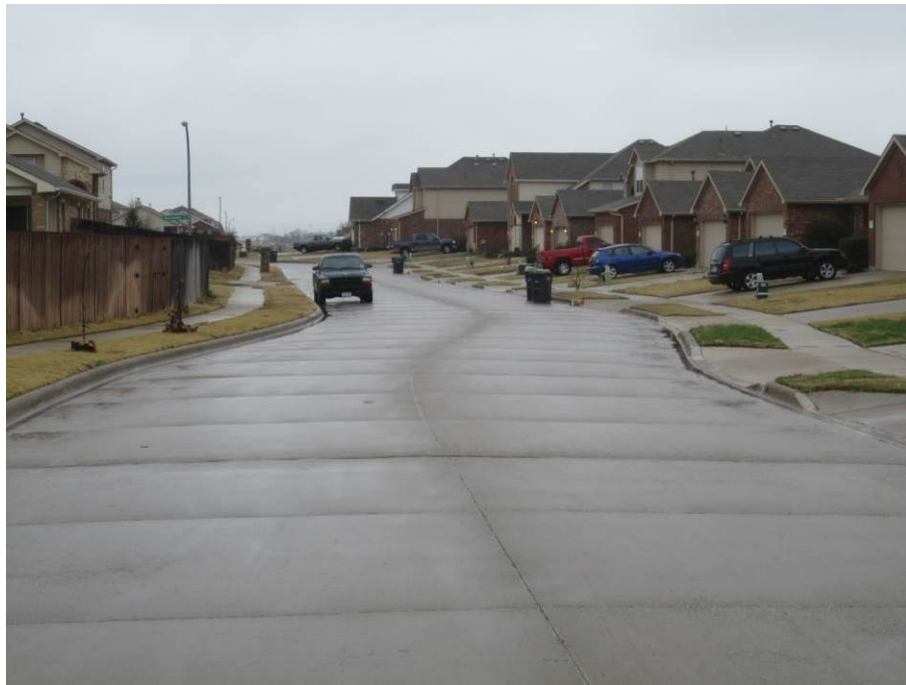
Figure 33. Alexandria Meadows subdivision streets constructed with ICC.
