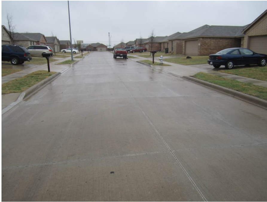
Figure 30. Residential ICC pavement constructed in 2005 at Windsor Park.
