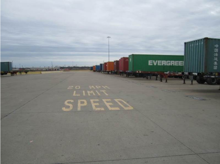
Figure 23. ICC pavement at UP Intermodal Terminal.
