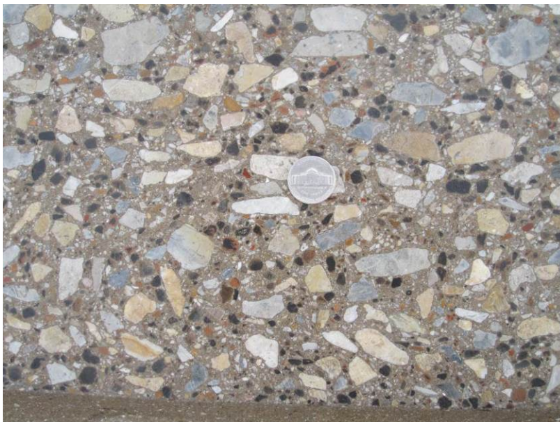
Figure 35. Close-up of ground-off surface of ICC concrete at Alexandria Meadows.
