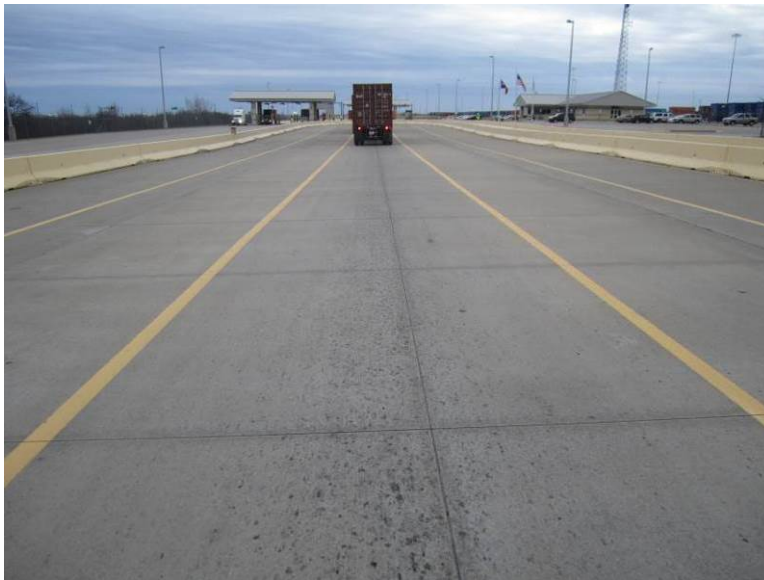
Figure 25. Heavy truck container entrance/exit traffic lane at the UP Intermodal Terminal.
