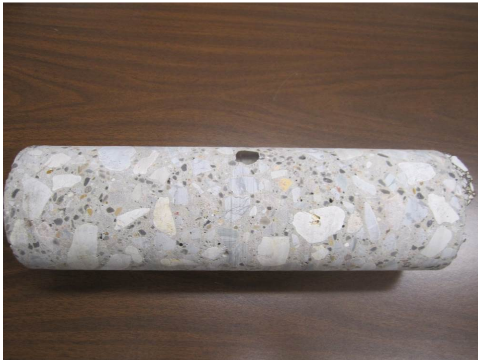
Figure 10. Close-ups of core taken from SH 121 CRCP from the ICC section. Note the small dark lightweight aggregate pieces throughout the concrete.
