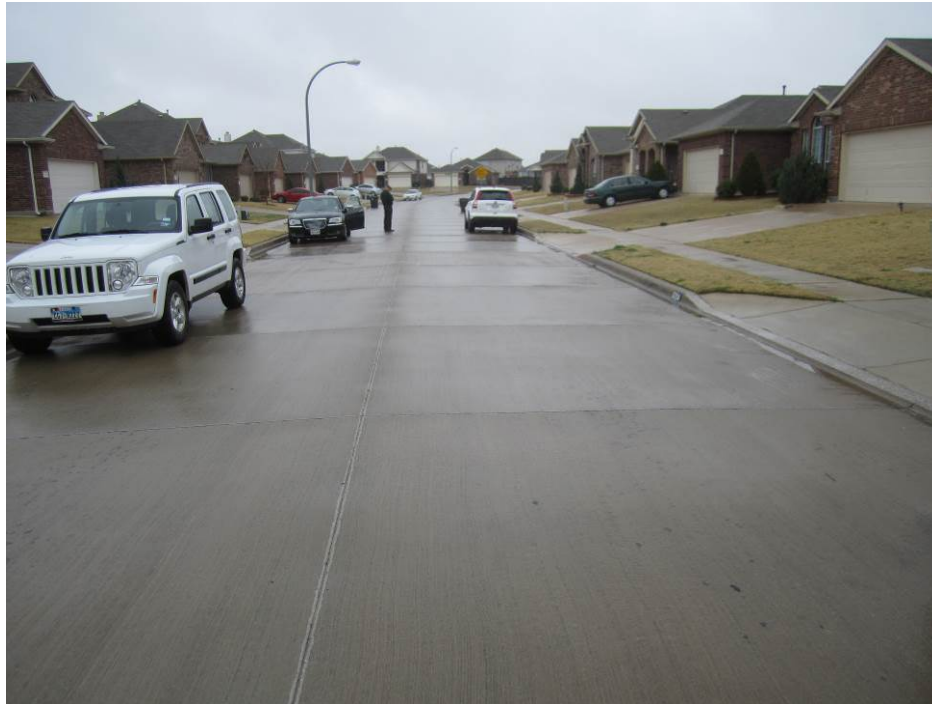
Figure 34. Conventional concrete streets built in Alexandria Meadows at about the same time (2005-2006).
