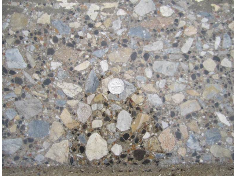
Figure 32. Close-up of ground-off surface of ICC at Windsor Park subdivision.
