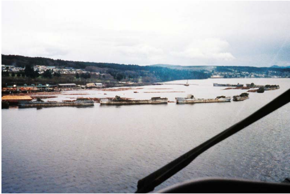
Fig. 1 Aerial view of the ten concrete ships at the Powell River site. (Photograph compliments of Tom Holm, Expanded Shale Clay and Slate Institute).
