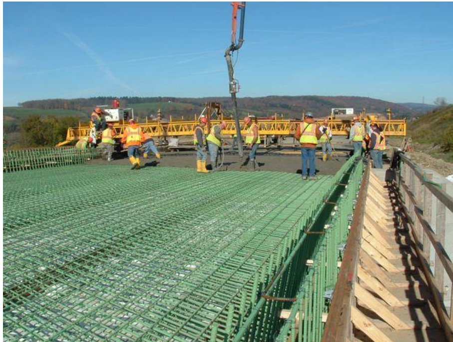
Figure 2 – Placing ICC on Interstate 81 over East Hill Road
