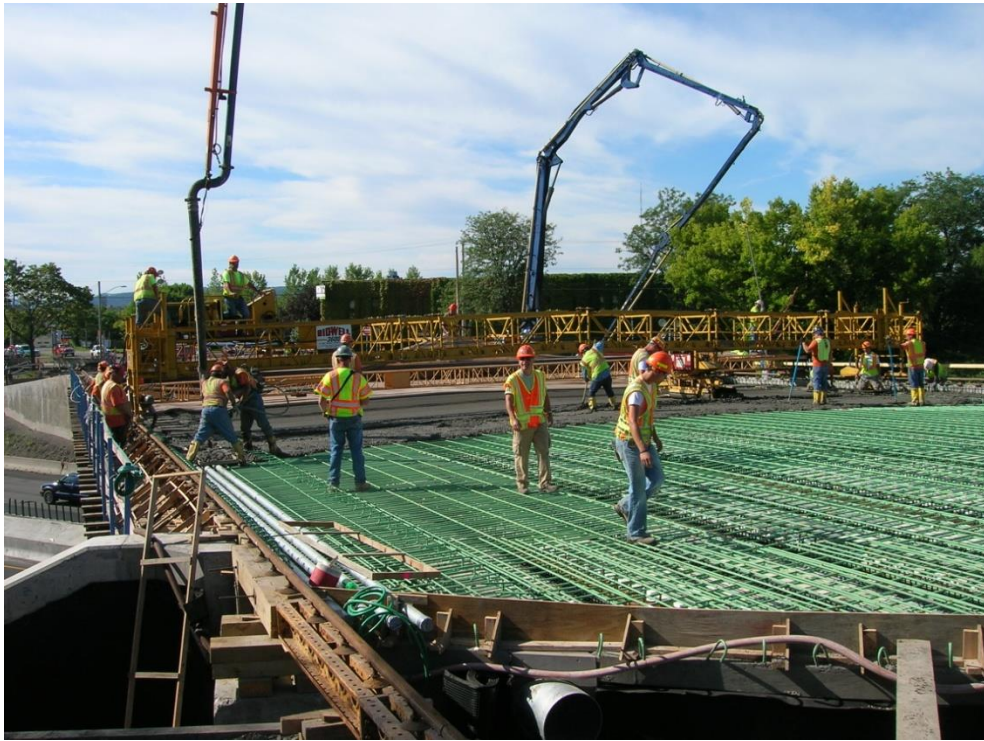
Figure 3 – Court Street Deck Placement
