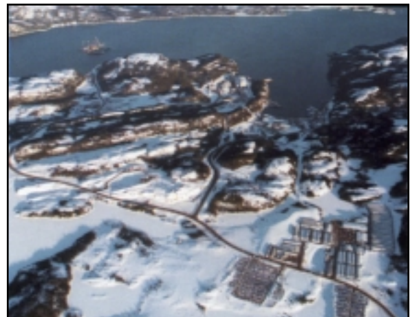
Remote construction site, Bull Arm, Newfoundland
