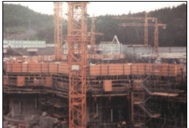
View of the massive, heavily reinforced “ice walls”
