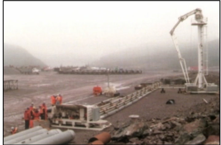
Pumping trials for long distance, high pressure, high workability concrete
