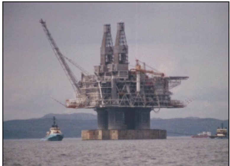
Completed platform being towed to Hibernia Oil Field site in the North Atlantic
