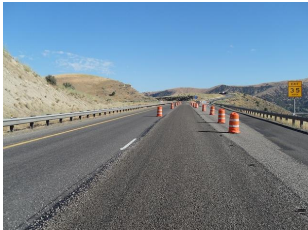
LWA Chips being applied over an existing LWA chip seal that was applied in 2004 on I-80 near Coalville, UT. Picture taken in August 2010.
