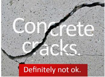
Since concrete cracking is most often the result of overt shrinkage, the life of concrete can be severely reduced as early age cracks grow in size. Cracks weaken the concrete by exposing its insides to many deleterious things from its in-situ environment. Over time, concrete cracks become exacerbated as small cracks grow into larger cracks.
