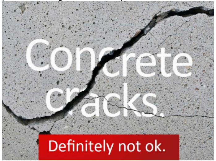
Since concrete cracking is most often the result of overt shrinkage, the life of concrete can be severely reduced as early age cracks grow in size.
