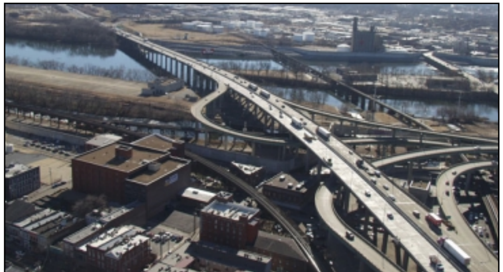
Northbound view of James River Bridge in Richmond, VA
