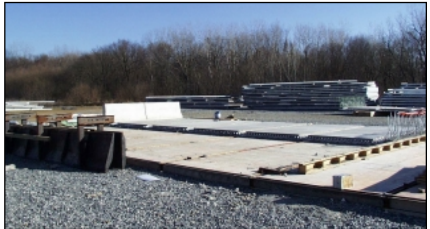
Span sections being fabricated and cured in casting yard
