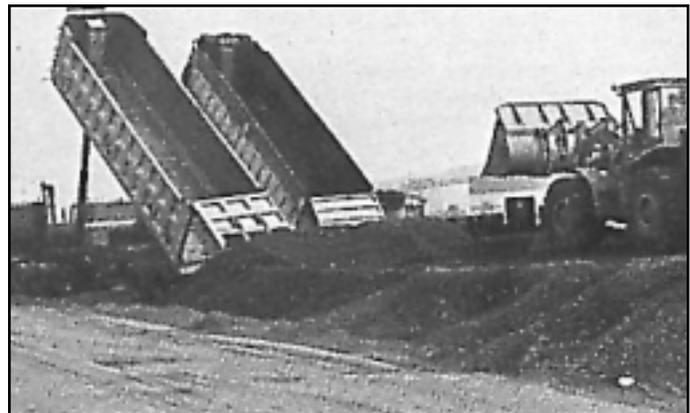
Fig. 4 Trucks dumping lightweight behind sheet piling wall
