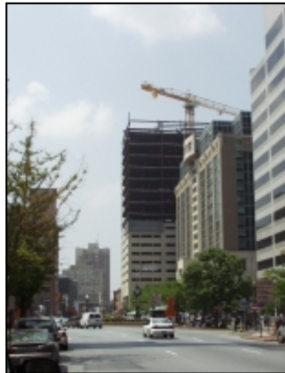
Market Square Plaza under construction
