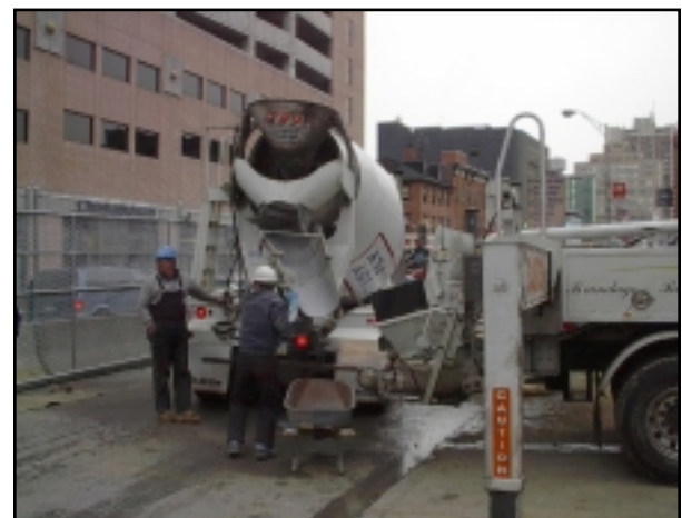
Pennsy Supply discharging concrete for lab testing
