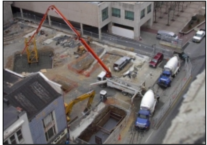
Pumping concrete for tower crane footer
