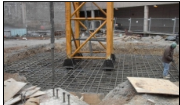
Tower crane footer and installation
