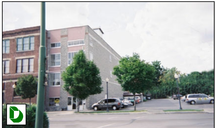
Rehabilitation of Emerson Building, Glens Falls, NY – 7,000 ea. 8” Smartwall splitface block
