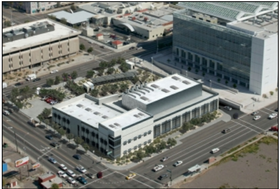
Aerial view of Phoenix Crime Lab, Phoenix, AZ
