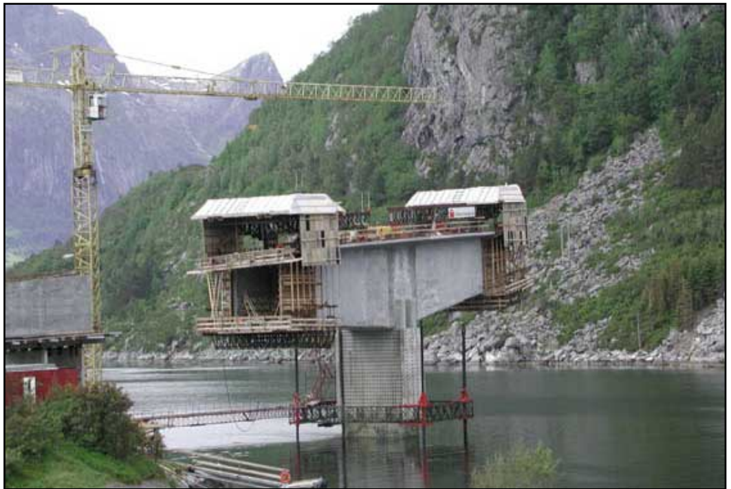
Cantilevered main span of Rugsundet Bridge under construction
