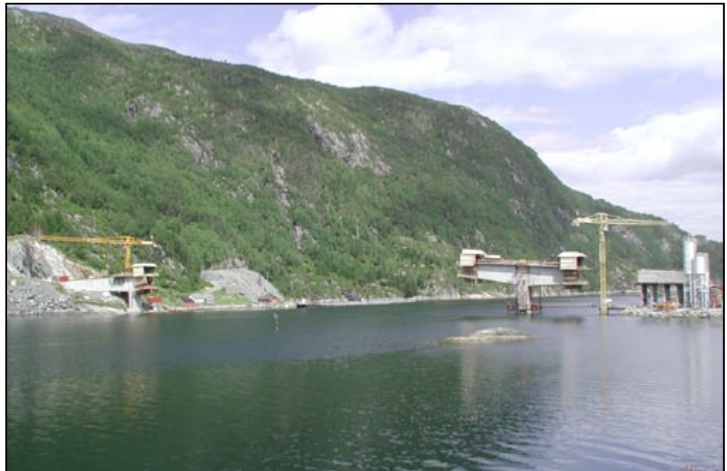
Rugsundet Bridge Under Construction
