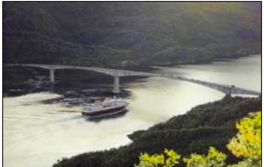
Completed Raftsundet Bridge
