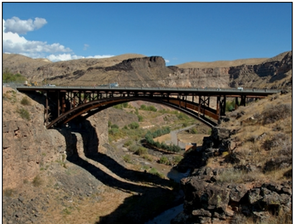
Virgin River Bridge, Hurricane, Utah
