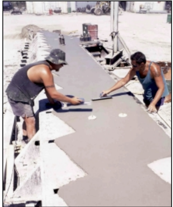
Bottom ranker element being finished in precast plant
