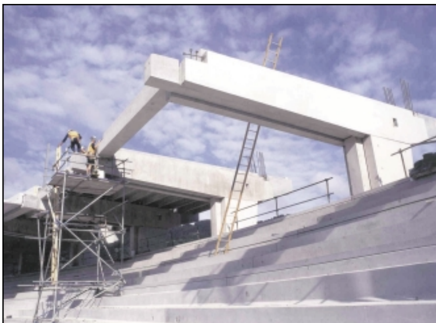
Cantilevered precast roof support with connecting precast cross member being secured.
