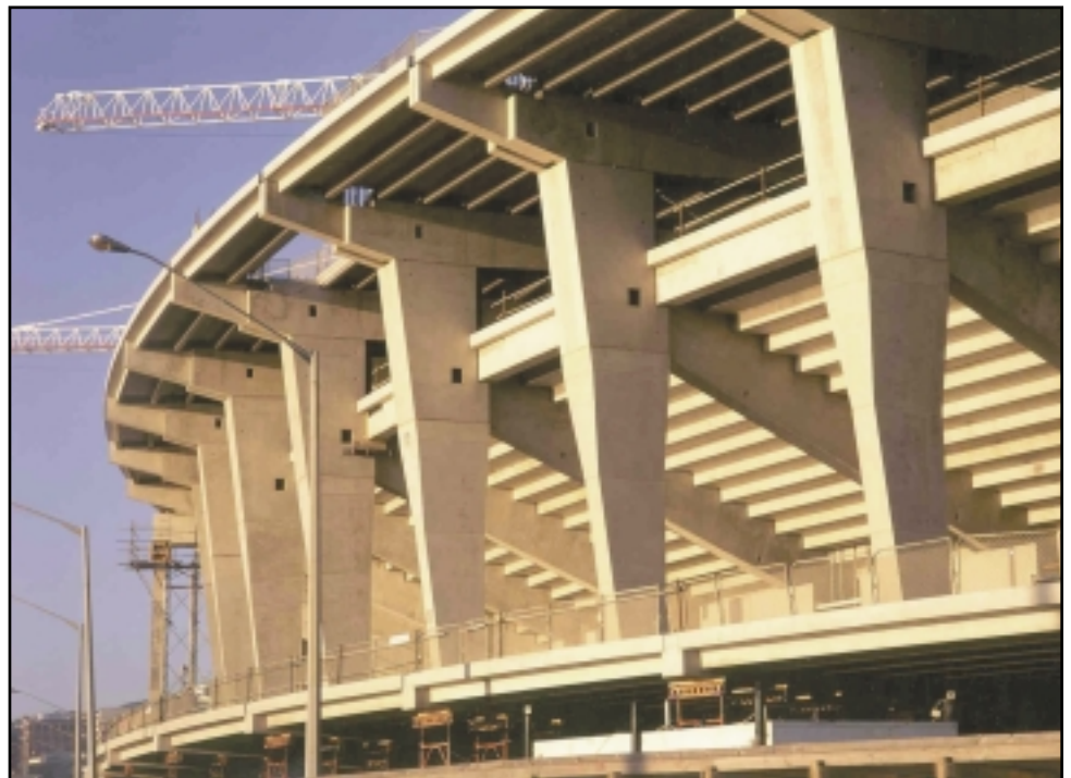
Exterior of 40,000-seat Wellington Stadium nearing completion
