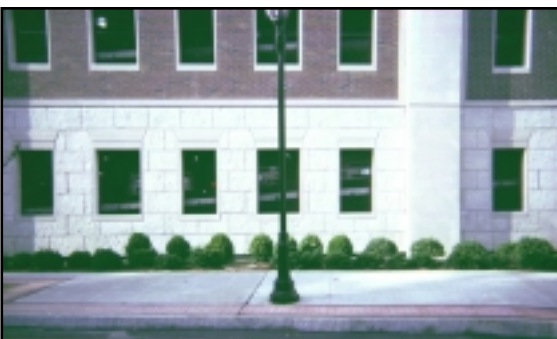
View of parking structure from Martine Ave.
