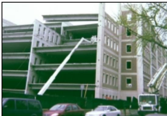
View of parking structure from Martine Ave.
