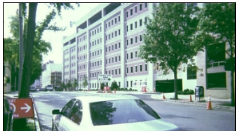
View of parking structure from Martine Ave.
