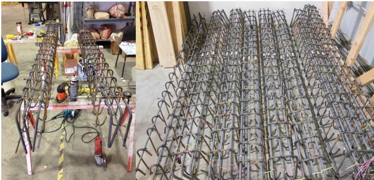
Figure 5-13- Fabrication and instrumentation of reinforcing cages
