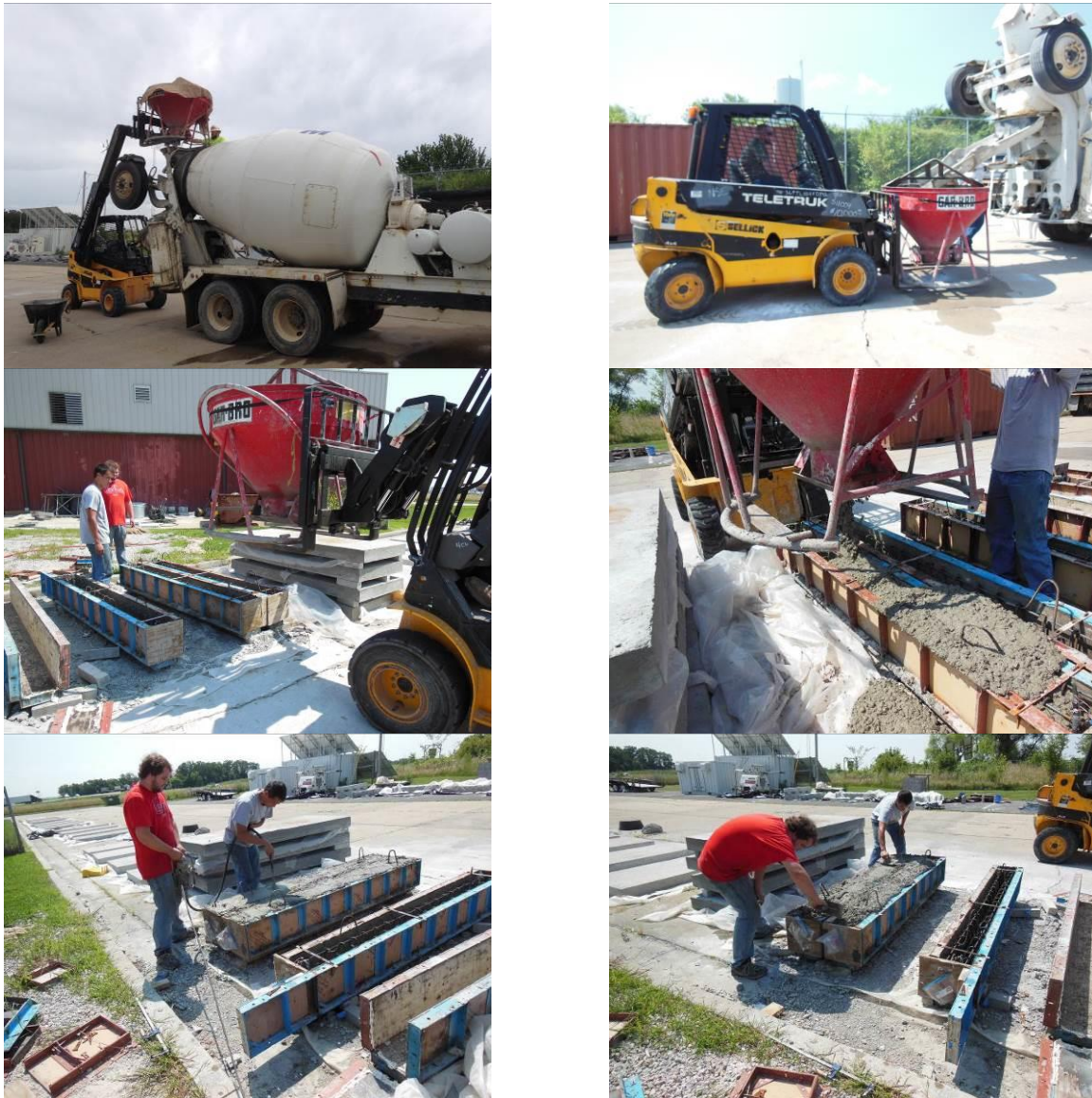
Figure 5-17- Concrete beam construction procedures
