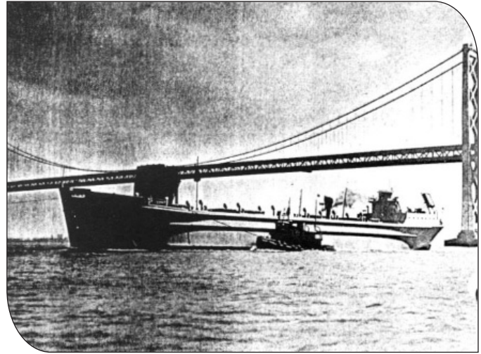
Figure 2. Concrete ship passing under San Francisco-Oakland Bay Bridge. Both ship and bridge made extensive use of lightweight concrete (ESCSI 1971).
