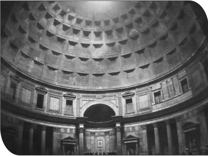
Figure 1. The Pantheon's dome consists of lightweight concrete that spans over 43 m (142 ft).
